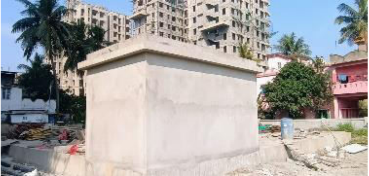
UNDER-GROUND WATER RESERVOIR
