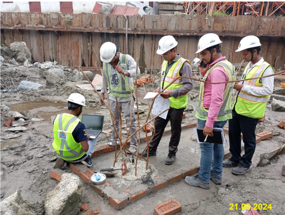
Pile Integrity test is in progress
