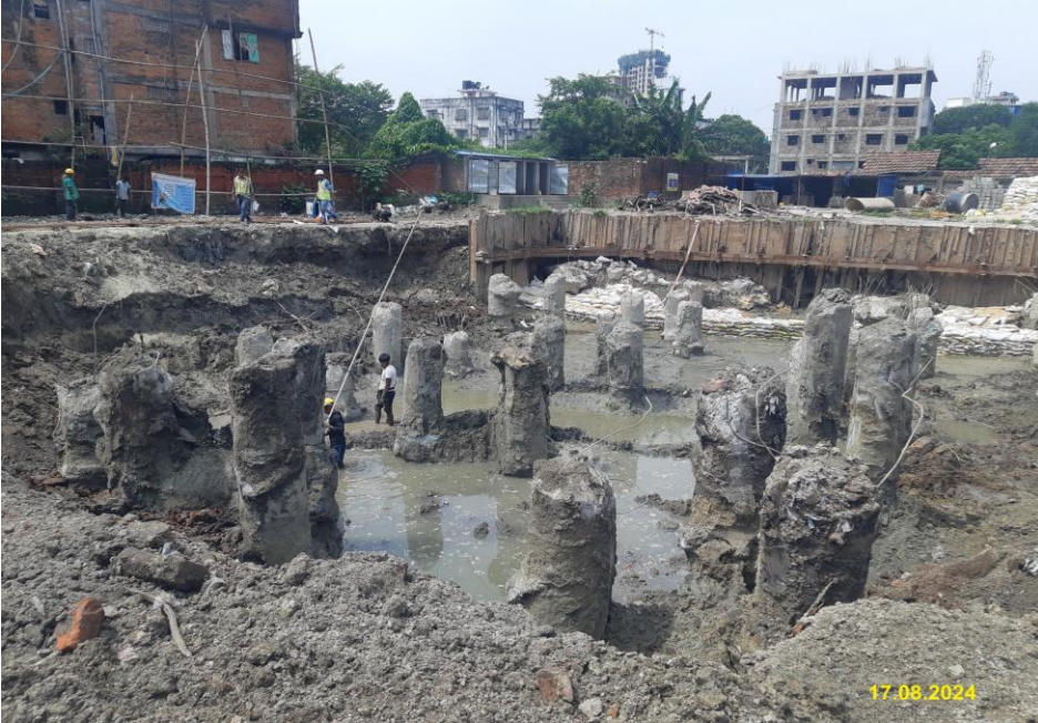
Pile Head Breaking is in progress
