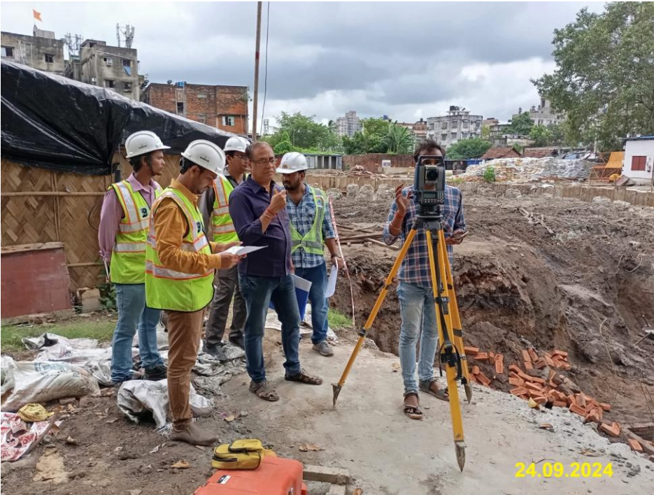
Block Layout checking is in progress
