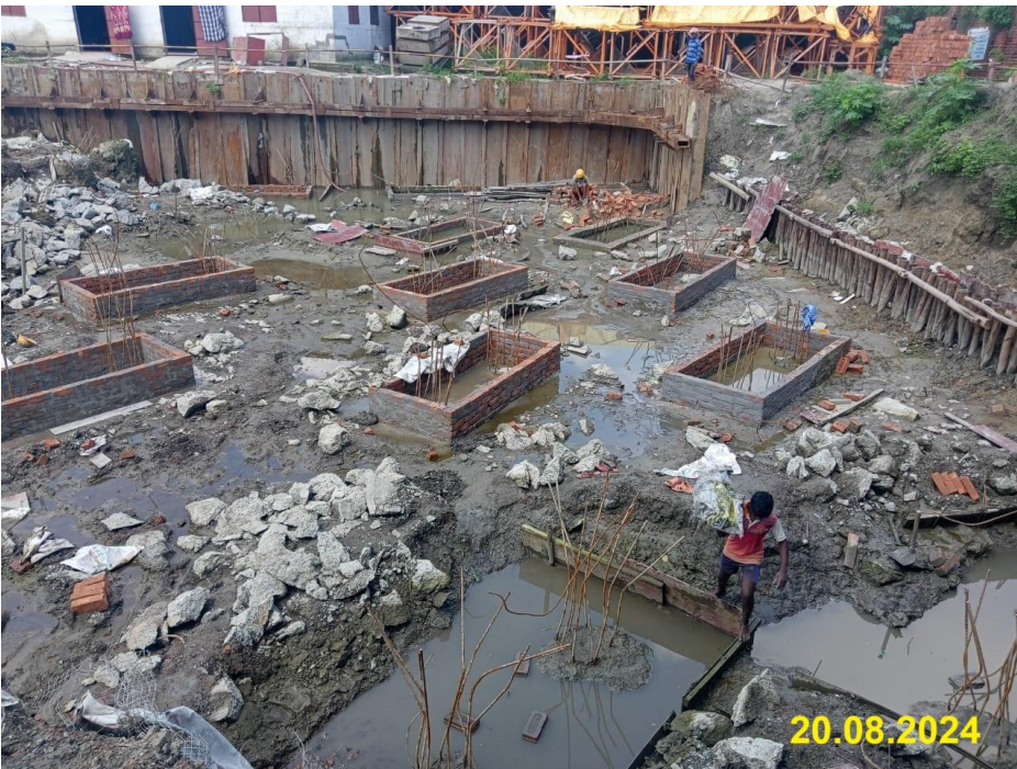
Pile Cap PCC work is in progress
