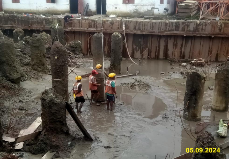
Pile Head Breaking is in progress
