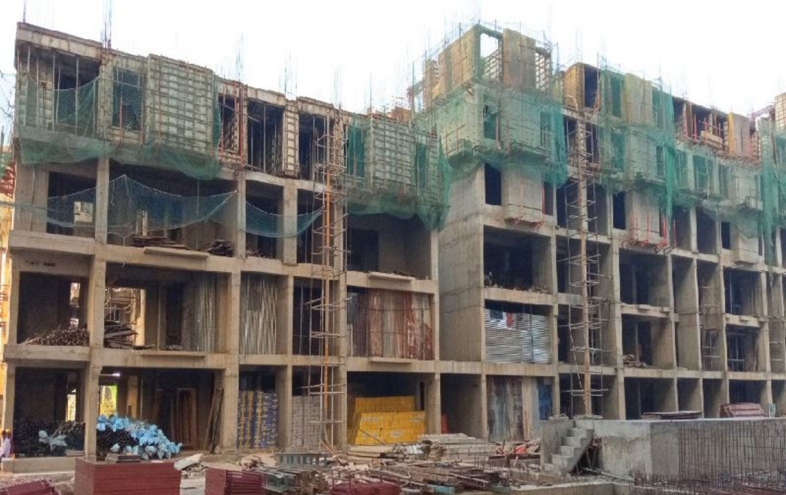
TOWER-5 (A) :: 3rd & 4th Floor Roof in progress
