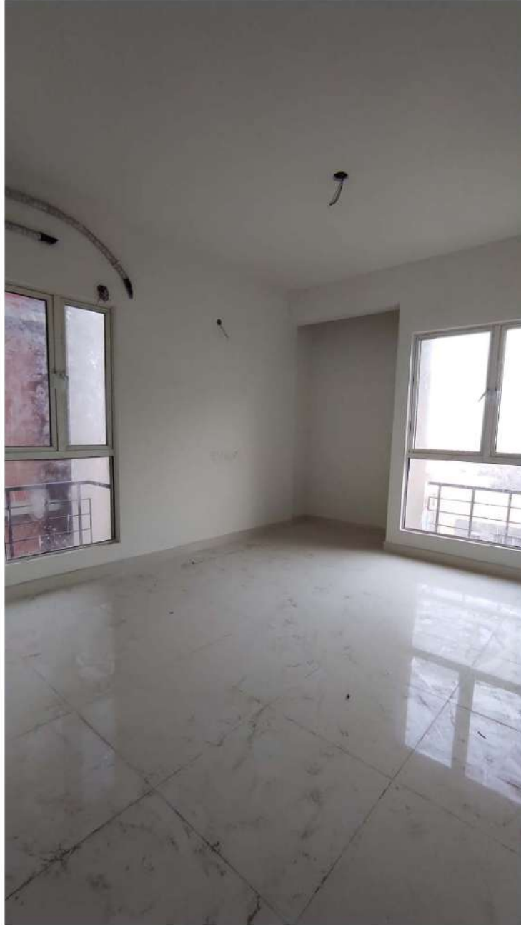
Block 2 & 3 Flooring Completed
