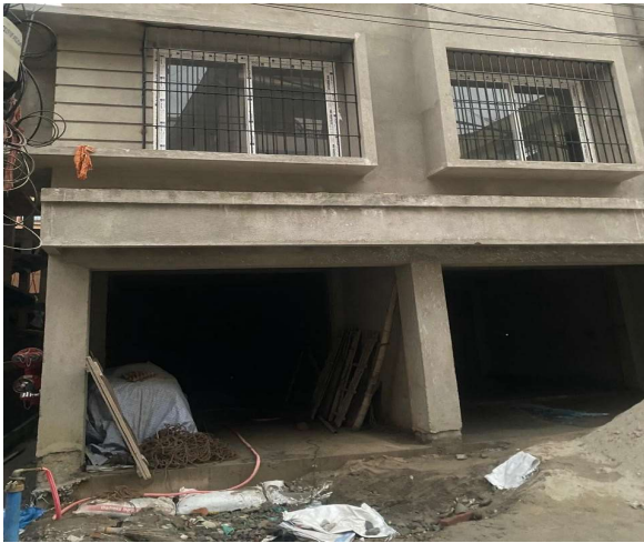
1 Shop- Under Process
